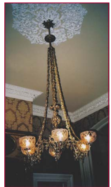
Retrofitting to resemble gas lights with fibre optics
