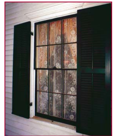
Window restoration at Knott House
