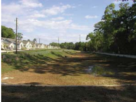
Large total retention facility at Camp's Crossing
