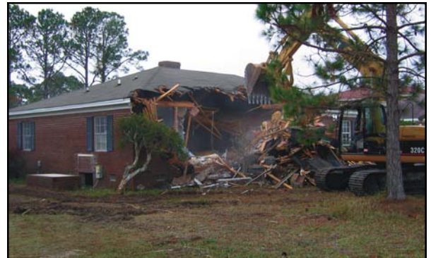
Home being demolished due to mold from water damage
