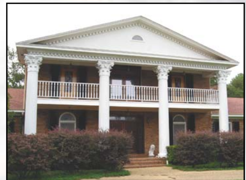
Tallahassee home protected by Hurricane Shutters
